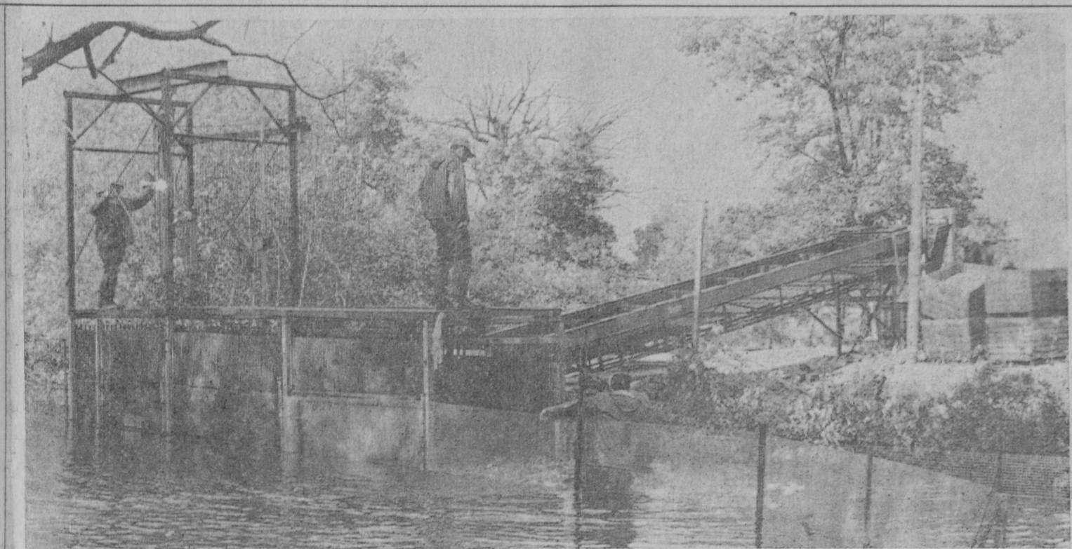
Coho salmon were herded into this collection area and conveyor lift system in the Tawas River.—Tawas Herald Photos.
