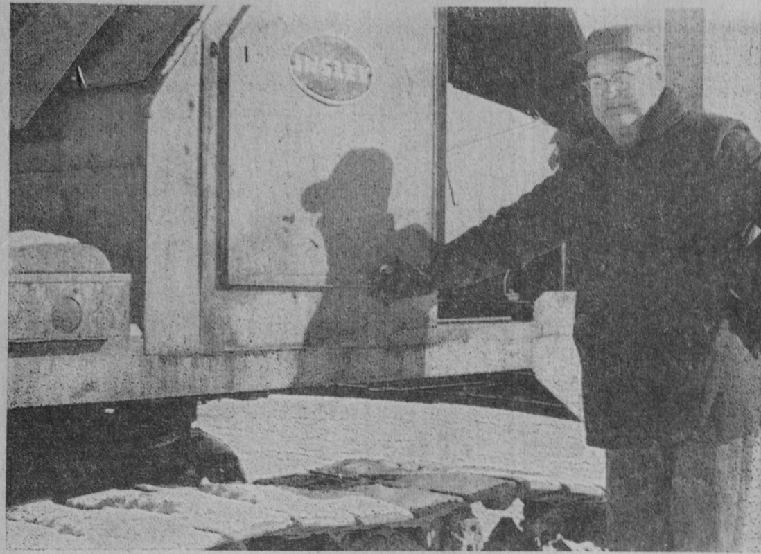
EDWIN ANDERSON takes a last look at a crane which he operated for the Iosco Road Commission before retiring Friday. He had worked 41 years for the commission.—Tawas Herald Photo.
