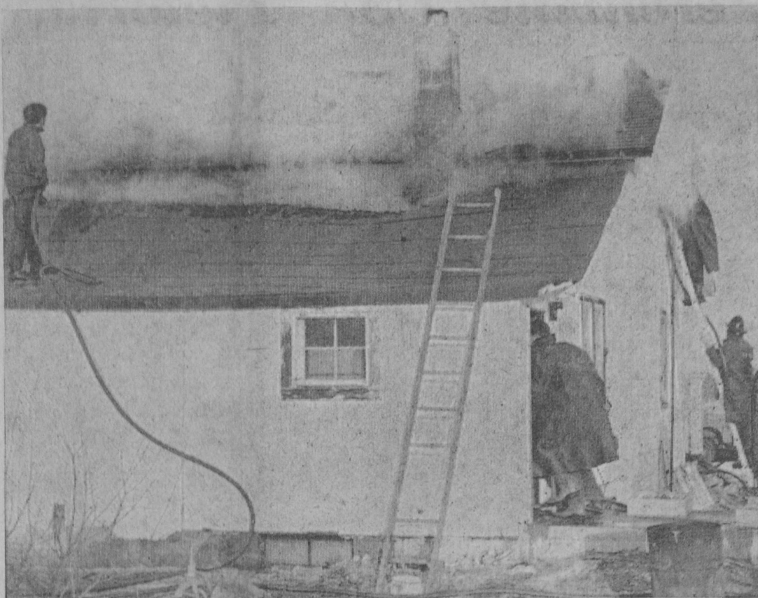
FIRE gutted the home of Mr. and Mrs. David Propper, Alabaster Township, Saturday afternoon. The family was not home at the time and there were no injuries. Tawas City firemen battled the blaze for a little more than one hour. Flames were in the attic and sidewalls. The house is owned by United States Gypsum Company and located on US-23.—Tawas Herald Photo.
