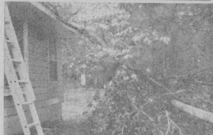
A FREAK TWISTER hit the Chain Lakes Road area between South Branch and Jose Lake last Thursday afternoon. Most of the damage was to trees. The Joseph Brandt home is pictured above showing the damage. The tornado was not sighted and unexpected, although hailstones fell for 15 minutes. Consumers Power Company crews worked all night to restore electrical service the next day at 8:00 a. m.—Pictures by Mrs. Joseph Brandt.
