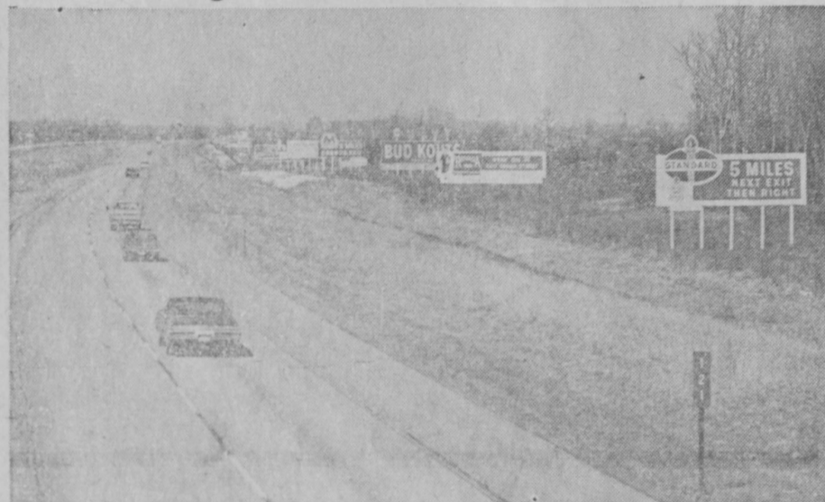
BILLBOARD ROW along Interstate 96 east of Lansing, first target of a move by the Department of State Highways and Attorney General's office to remove illegal billboards. Not all of these boards are illegal. Owners of those that are must remove them within 30 days. The Highway Department will move next against illegal billboards along I-69 and I-75. (Department of State Highways photo).
