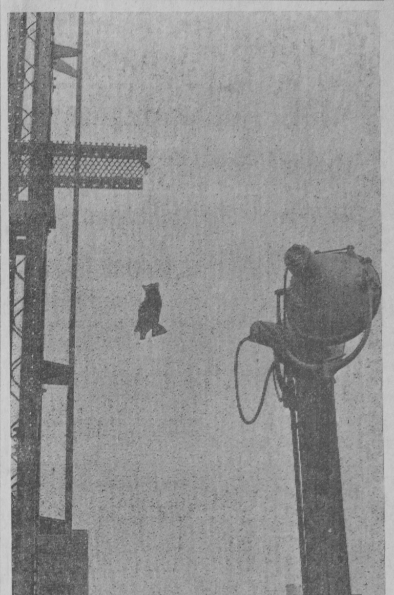
PROBLEM of starlings roosting and nesting in substations has long plagued the electric utility industry. A night-flying starling can fly into an electrical transformer and easily knock out the power for thousands of homes. A pair of Consumers Power Company employees have developed a method of frightening starlings away from substations. Borrowing a trick used by varmit hunters—only with reverse effects—the company is using decoy owls attached to nylon cords, to frighten the starlings away. At night, a timer-operated flashing light does the same job.
