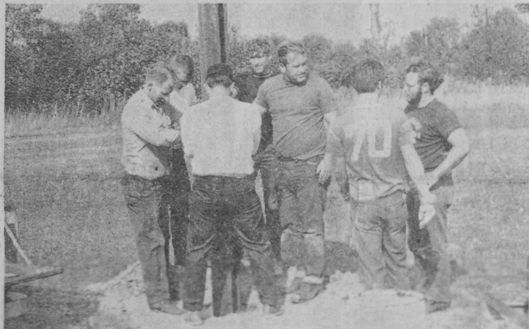
INSTALLATION of a new scoreboard started last week at Hale Area High School's lighted athletic field. The scoreboard was purchased by the class of 1971 and installation is being completed by volunteers from the community. Lights for the field were purchased through a fund-raising drive by the Hale Lions Club.—Tawas Herald Photos.
