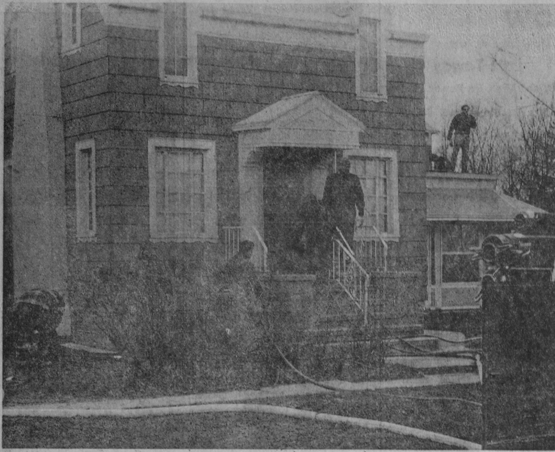
EXTENSIVE DAMAGE was caused to the home of Mr. and Mrs. Fred Brabant of Second Street, Tawas City, Monday afternoon. Firemen believed that faulty electrical wiring caused a blaze near a clothes drier. Flames burned through the kitchen wall, an upstairs bedroom and the north
