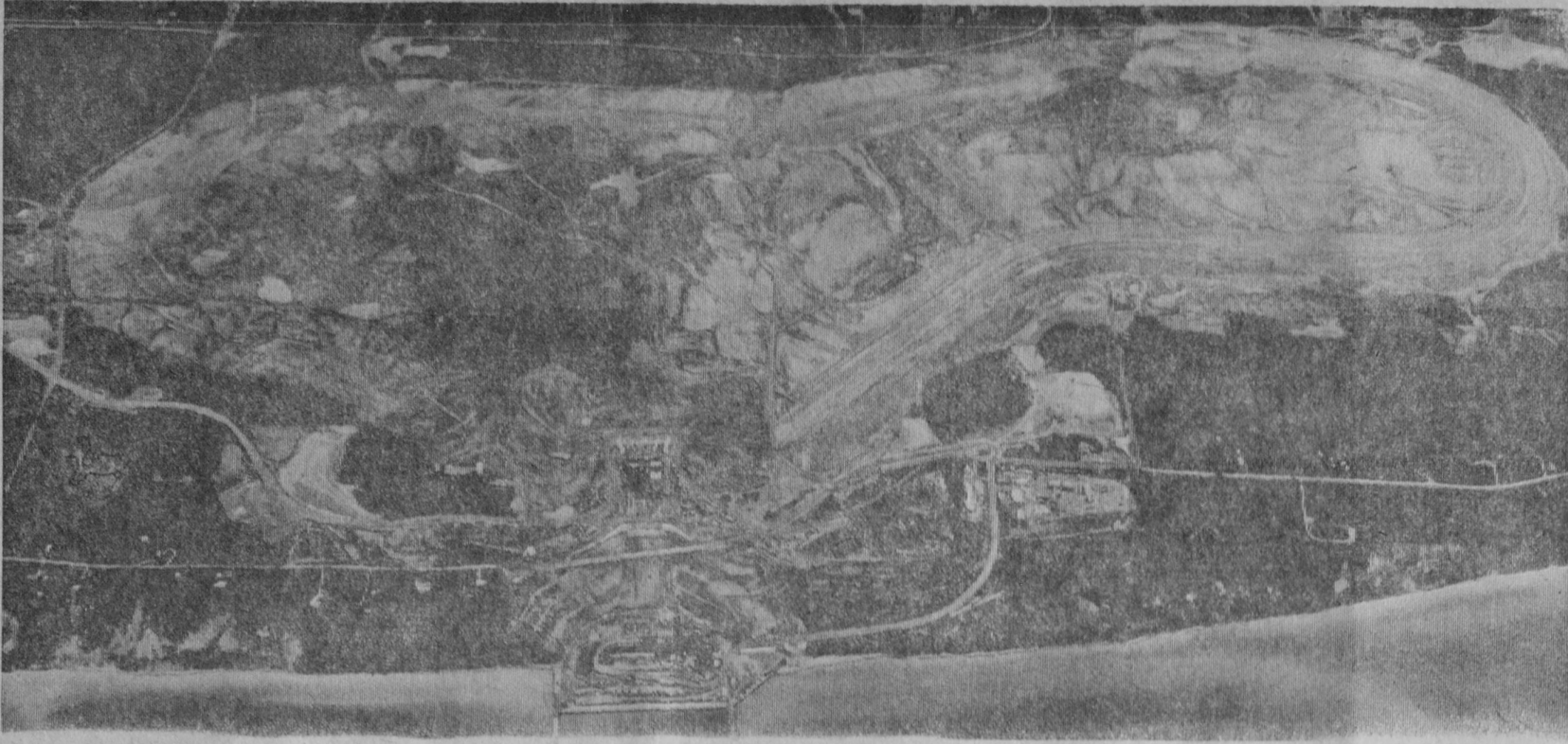
THE LUDINGTON pumped storage hydroelectric plant (above) is being constructed by Consumers Power Company and Detroit Edison Company to have a minimal effect on the natural environment of the area. The facility, located on Lake Michigan four miles south of Ludington, is scheduled for completion in 1973.
