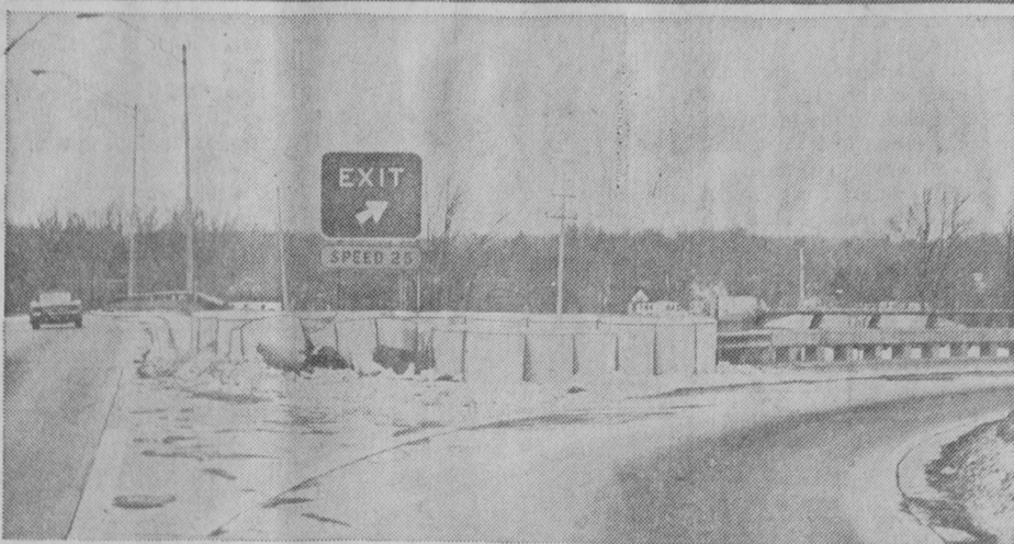
DOING THE JOB — Clusters of plastic barrels, partially filled with sand, are proving effective in preventing serious accidents at several exits on Michigan freeways. Top photo shows vehicle crashing into barrels at high speed. Below is aftermath of collision at I-496 Freeway exit in Lansing. In seven accidents at this site, drivers have been able to back off and continue on. (Department of State Highways photo)
