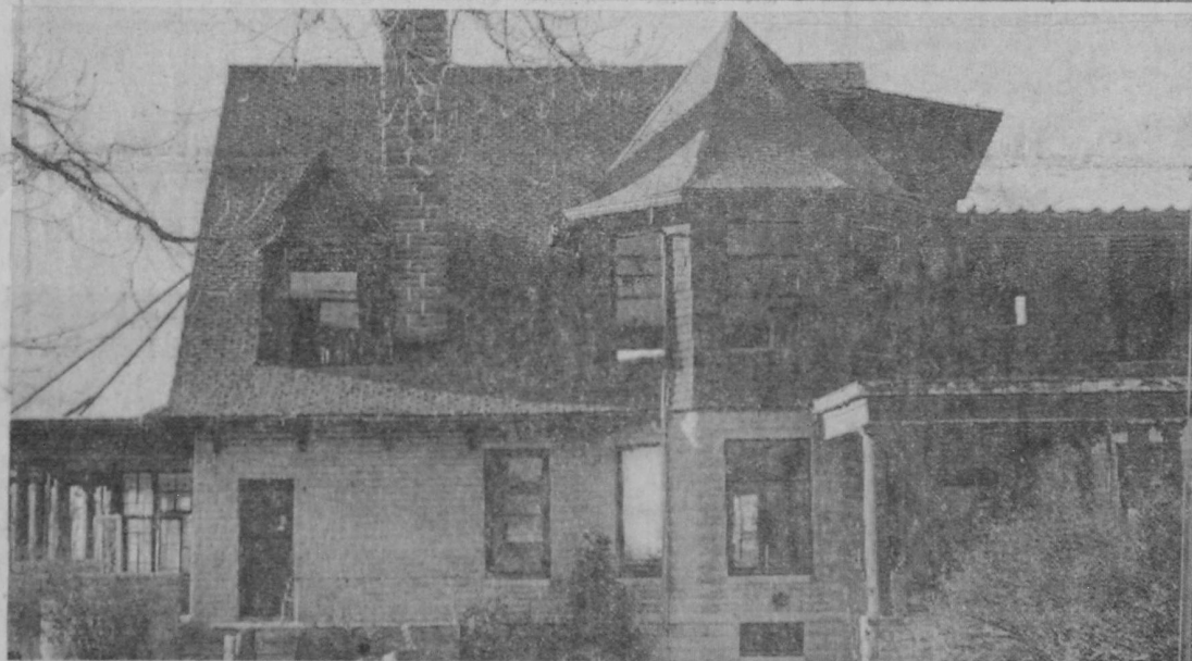
CALLED "one of the most handsome homes in this section of the state" by the Herald editor when it was nearing completion in October 1905, the residence of G. A. Prescott, then secretary of state, is in the last stages of being razed. The 66-year-old landmark at the corner of Lake and River Streets was constructed at the end of the lumbering era. The family's mill was destroyed by fire that year and, although still operating a large store in Tawas City, the Prescotts were beginning to concentrate on the raising of sheep at their farm in Ogemaw County. The residence was one of the first in Tawas City to be lighted electrically. The property, owned by Dr. and Mrs. J. D. LeClair since 1952, is being cleared for commercial purposes.—Tawas Herald Photos.
