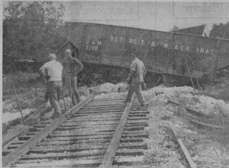
A SPLIT RAIL in the Detroit and Mackinac Railway's track early Thursday morning caused a massive derailment north of East Tawas. Members of the Tawas shop crew assisted section workers in clearing tracks of twisted cars and debris in order to open the line to traffic by Friday noon. Edward Goodman, president and general manager, said the wreck was still under investigation. Thirteen cars were derailed and damage is to be estimated as soon as all cars are returned to the Tawas yard. There were no injuries in the wreck, although the two-engine unit, with Richard Nowak of Alpena as engineer, passed over the defective rail and the first car was thrown off the tracks. Work on clearing the wreckage is pictured here.—Tawas Herald Photo.
