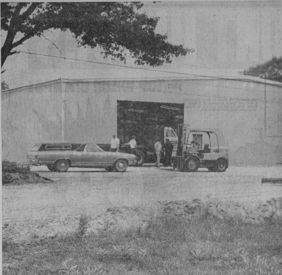
WORK was completed this week on Schreck Lumber Company's new warehouse. The 100 by 200-foot all steel building is fully insulated and will be used for storing plywood, roofing and insulation. A pre-inventory sale is being held this week as materials are
