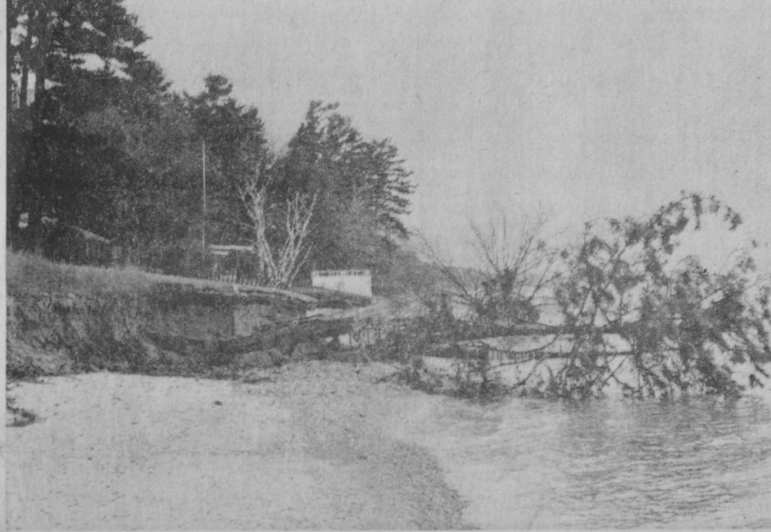
IOSCO'S SHORELINE along Saginaw Bay was not hit as hard as the shoreline of Bay County and Arenac County in last week's storm, but there was considerable damage to seawalls from the county line north through Alabaster Township. These pictures were snapped in front of the Bernard A. Stelter Jr. residence on Douglas Drive south of Tawas City and show the effect of the storm on a seawall protecting his property. Wave action
