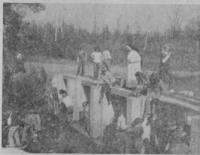
This dam was inspected at the Rifle River Recreation Area.
