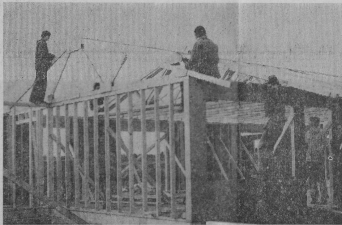
STUDENTS are shown installing rafters which they designed and constructed for the house. Some 21 boys are participating in this project. Materials and financing are being provided by
