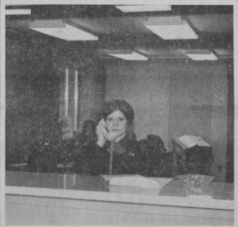
WORK IS PROGRESSING on remodeling former living quarters into offices for the sheriff's department. The new main office facing US-23 was used for the first time last week. Denise Heari, clerk, is at the telephone.—Tawas Herald Photo.
