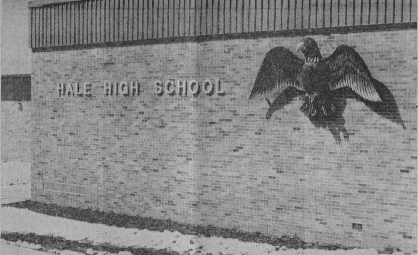
A LARGE FIBERGLASS EAGLE, emblem of Hale Area School, was installed on the south wall of the new Hale Area High School Thursday by Powers Aluminum. Donated to the school by Douglas Powers, the three dimensional eagle measures 11 feet by six feet.—Photo by John Sherer.
