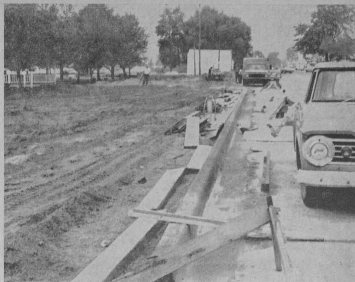
CONTRACTOR for the City of Tawas City is now engaged in a race against time to complete concrete work for a new parking lane and sidewalk along US-23 at the city park. Two delays, the first being a permit necessary from the state highway department for moving two electrical poles and the second being delayed shipment of steel forms for constructing concrete curbs, has
