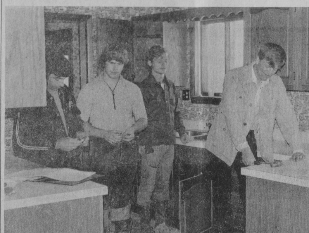
MAKING PLANS for completing the plumbing project on the house are, from left, Jerry Eno (instructor), Steven Anschuetz, Rick Ashmore and James Lewis, all members of the shared-time building trades program. Twenty-one students from four county high schools participated in the program.—Tawas Herald Photo.
