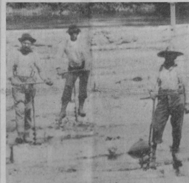
DEVELOPMENT of a new method of log rafting provided a practical means of towing saw logs from Georgian Bay across the wide expanse of Lake Huron to East Tawas and other manufacturing centers along the shore. These men are using long augers to bore holes through logs. A "bracelet" was formed by chaining the logs together and hundreds of logs floated in the enclosed area.
