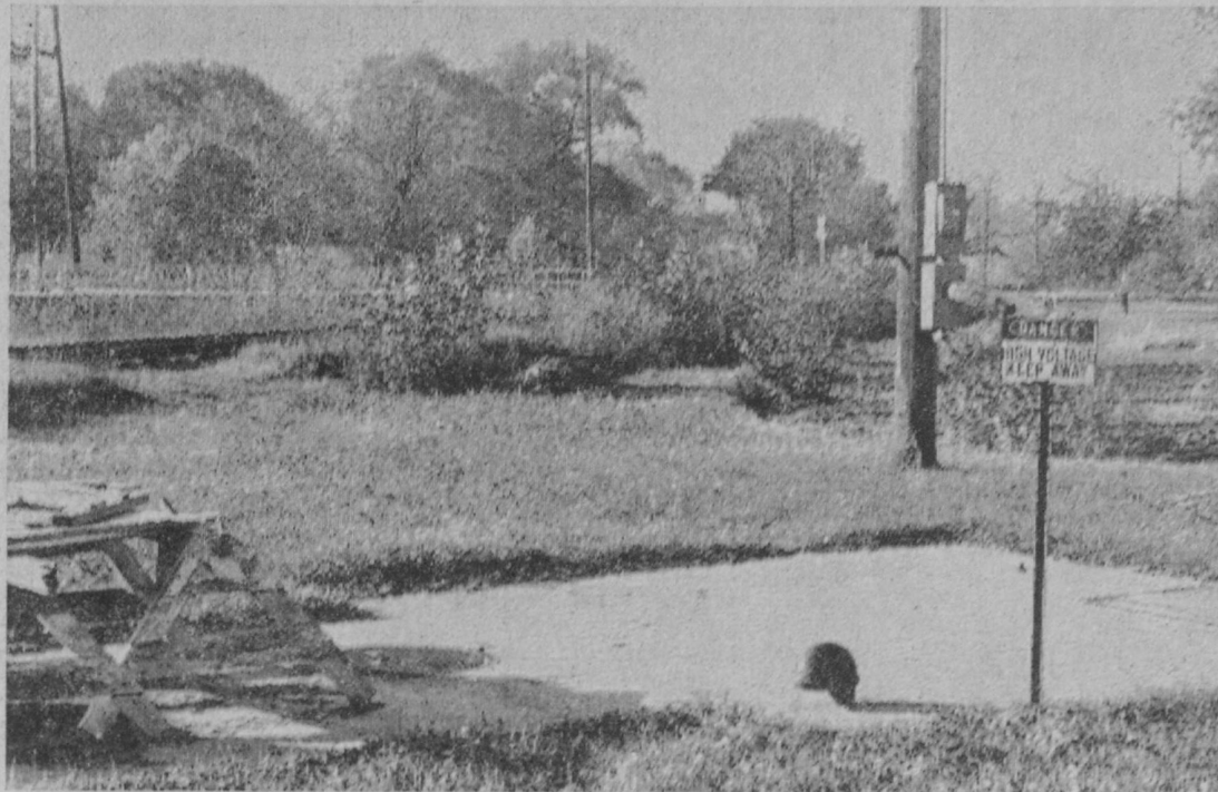
NOT AN IMPOSING STRUCTURE, but an important one to Tawas City's sewage disposal system. The concrete slab in the foreground covers a lift station on Second Avenue. Voters are
