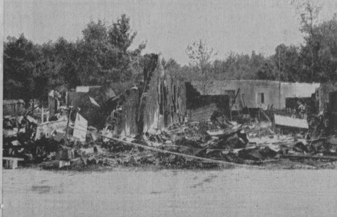
THE FLAMING WRECKAGE of the motorcycle and car then traveled nearly 300 feet and crashed into the former McIvor store and post-office, completely demolishing the old frame structure. Ruins of the building are shown here. —Tawas Herald Photo.
