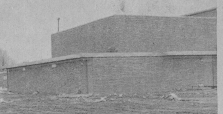
RESIDENTS of Whittemore-Prescott Area School District will take their first look tonight (Wednesday) at the new 10-classroom middle school addition which has been under construction since late summer. Parents and others interested in the school are invited to attend the regular meeting of the Whittemore-Prescott Parent-Teacher Association. An official open house is to be held in May. The $500,000 expansion program, added to the north side of the high school, also houses an expansion to the multipurpose room, a gymnasium, library, art room, general offices and rest rooms. Junior high school students moved into the new structure last week. The large library awaits completion in May. The top picture shows the exterior of the classroom addition. The smaller picture shows the gymnasium addition. Gene Gillette, director of special education, is shown with Mrs. Raymond Dorsey in the new administration office. A seventh grade class with Mrs. Jean Klinger, instructor, is shown in the lower photo.—Tawas Herald Photos.
