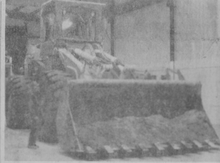
AFTER a 70-ton tractor rips through the gypsum seam, this huge front-end loader with a 10-yard "bite" scoops up the rock and loads it on the conveyer system.
