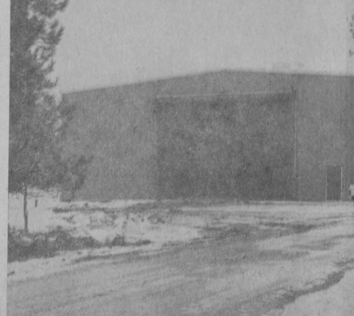
A NEW shop building and maintenance headquarters has been constructed west of Gypsum Road. The two-story building is large enough to accommodate the huge tractor and front-end loader with plenty of room to spare for work on other equipment.
