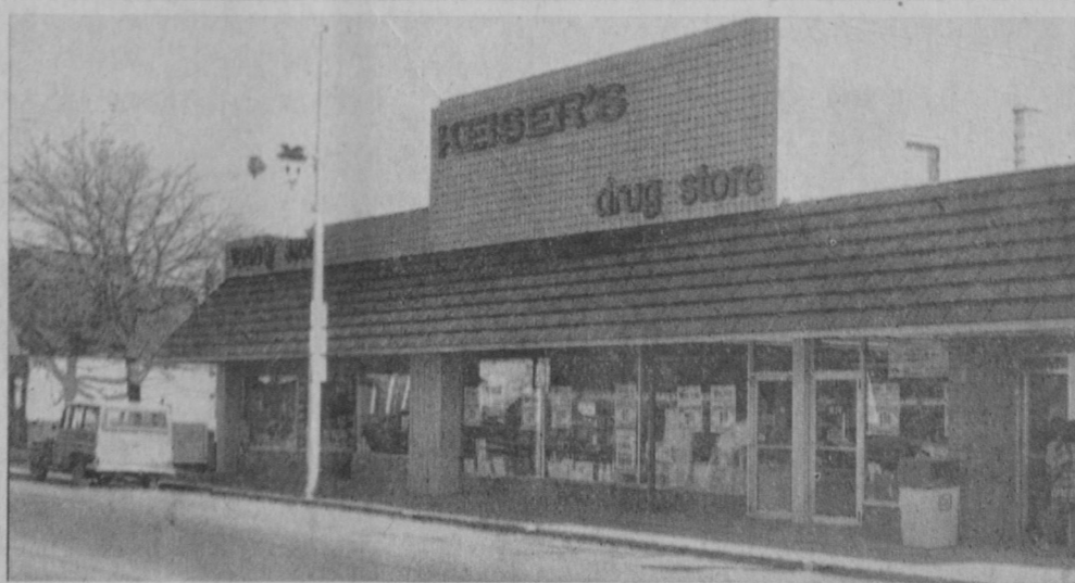
KEISER'S DRUG STORE in Tawas City, which this week observes its 50th birthday, is holding a golden anniversary sale. Turn to page 6, sec. 2, for holiday gift suggestions. The firm completed the remodeling of its building (above) earlier this year. —Tawas Herald Photo.
