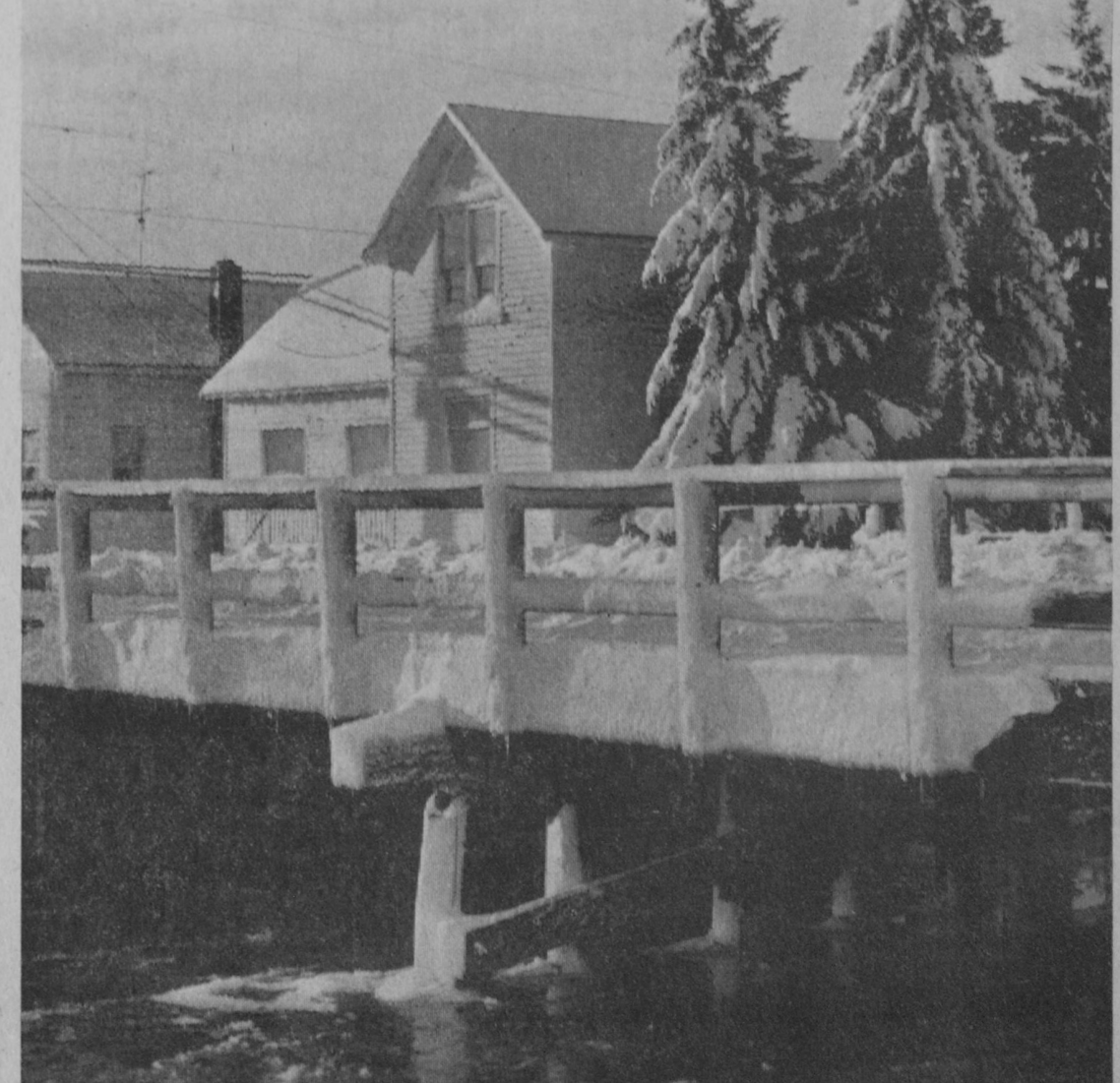
PRECEDING Thursday night's special meeting, members of the Tawas City Council will inspect the house shown directly behind the Mathews Street bridge to give consideration to purchasing the property for a public fishing site-purchase area. The house, one of the oldest structures in the community, was once owned by the late Mr. and Mrs. William Hatton. The property has been offered for sale to the city by the Federal Housing Authority.—Tawas Herald Photo.
