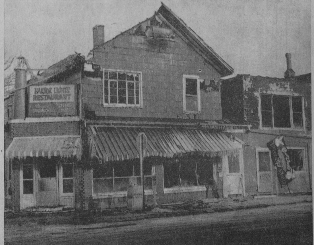
DAYLIGHT showed the Harbor Lights building, a frame and concrete block structure at the corner of Newman and East State Streets, in complete ruins. Only the shell remained after the six-hour blaze.—Tawas Herald Photo.
