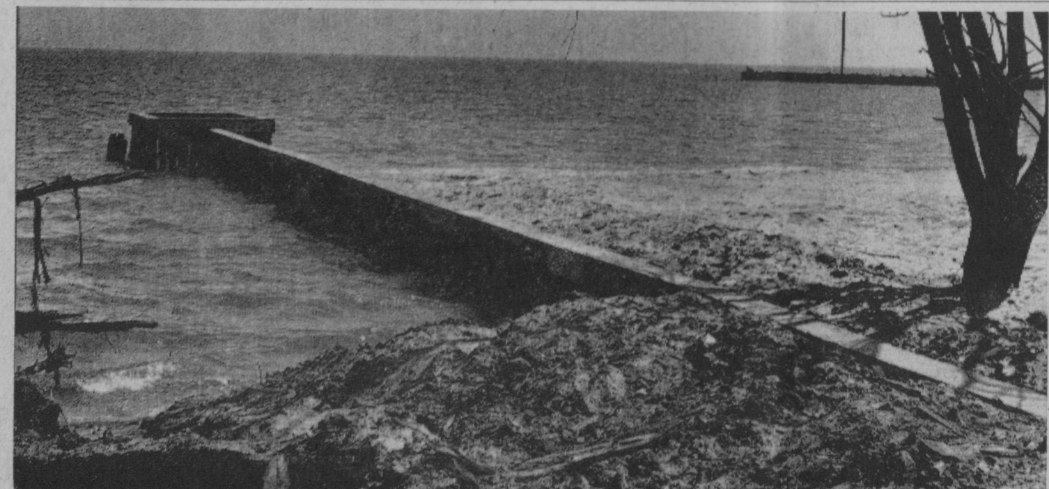
AN EXPERIMENTAL beach nourishment program conducted at the Tawas City Park by the Michigan Department of Natural Resources, in cooperation with the city council, appears to be an effective method of controlling shore erosion where littoral drift of sand is of a minor nature. The last segment of the project is construction of a groin extending into the bay from the east end of the park, which is to be completed this week. As the city's part of the cooperative project with the state, the groin is expected to provide a blocking force against littoral drift of sand
