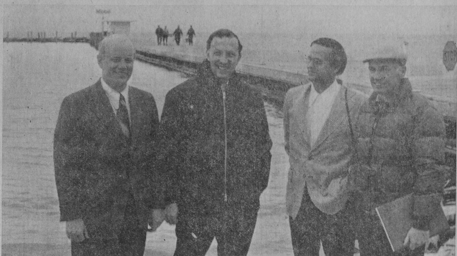
COMPILING INFORMATION to update plans authorized by congress in 1968 for a proposed extension to the Michigan Waterways Commission Dock is the United States Army Corps of Engineers and a Jackson consulting firm. Here last week to commence the study were, from left: Larry Everett, Fargo Engineering Company; George Platz, Detroit District, corps of engineers; Don Oliva, Fargo Engineering; Jack Collis, Detroit District, corps of engineers. The dock is pictured in the background.—Tawas Herald Photo.
