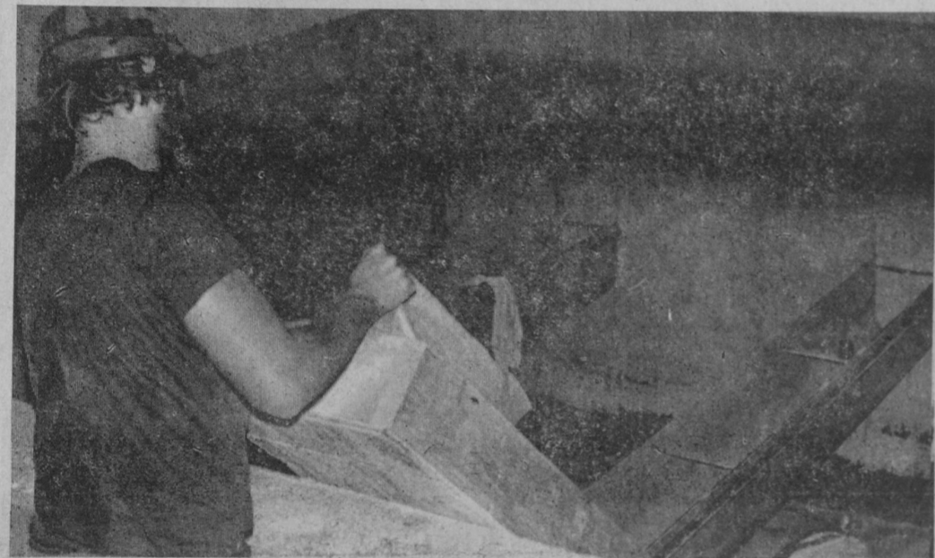
WORKMEN of Ames Construction Company, Saginaw, are shown here filling the filtration tank with 11 cubic yards of silica sand.—Tawas Herald Photos.
