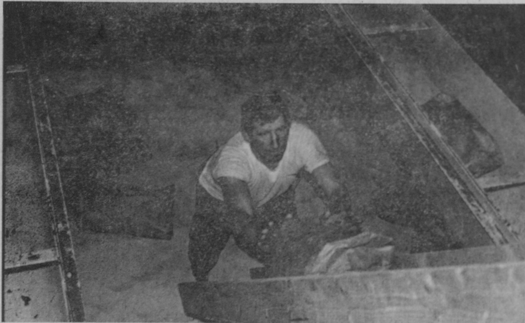
WORKMEN of Ames Construction Company, Saginaw, are shown here filling the filtration tank with 11 cubic yards of silica sand.—Tawas Herald Photos.
