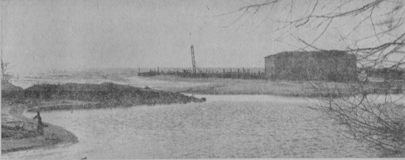
DRIFTING SAND has completely blocked the mouth of the Tawas River. Sand has closed the channel into Coho Marina, right, and
