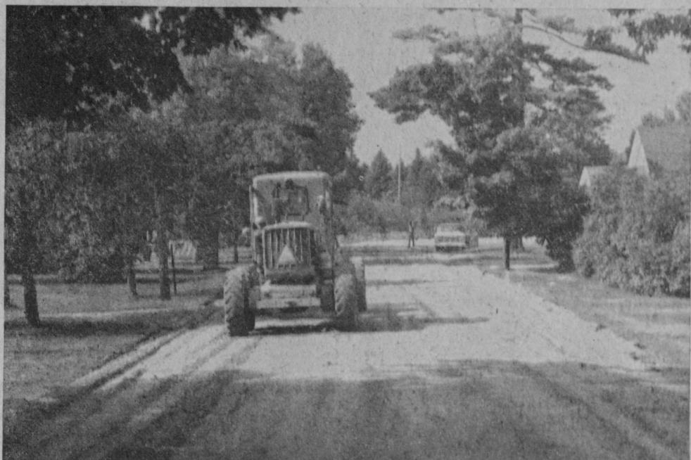
CREW and equipment of Tawas City Department of Public Works is preparing streets for blacktop work during the fall season. This picture shows a grader at work on River Street.—Tawas Herald Photo.
