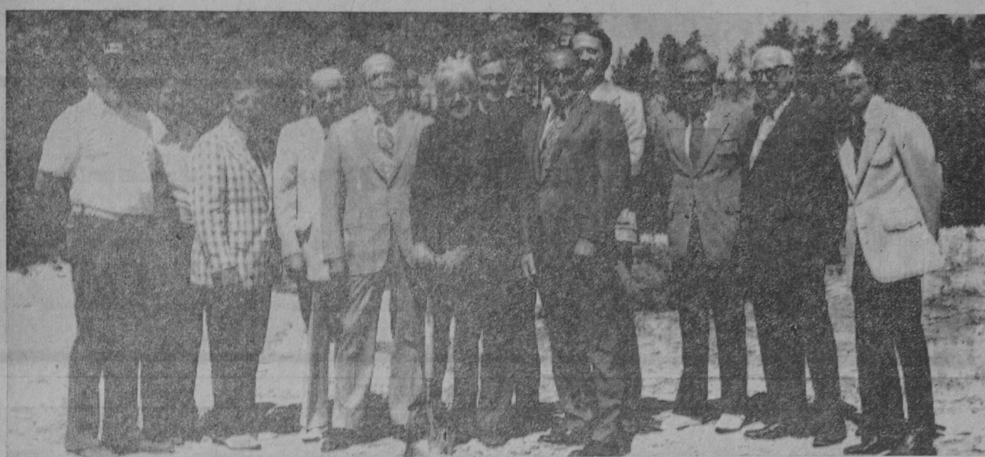
GROUND was broken Friday noon for McKay Sales Company's new salesroom and service center, to be located one mile east of East Tawas in Baldwin Center. The new one-half-million-dollar structure is to be completed in 1976. Watching L. G. McKay, center, breaking ground with a shovel are, from left: Edward Davison Jr., contractor; Mayor Robert Bolen of East Tawas; Roger McInosh, the firm's general manager; Richter Lixey, supervisor of Baldwin Township;
