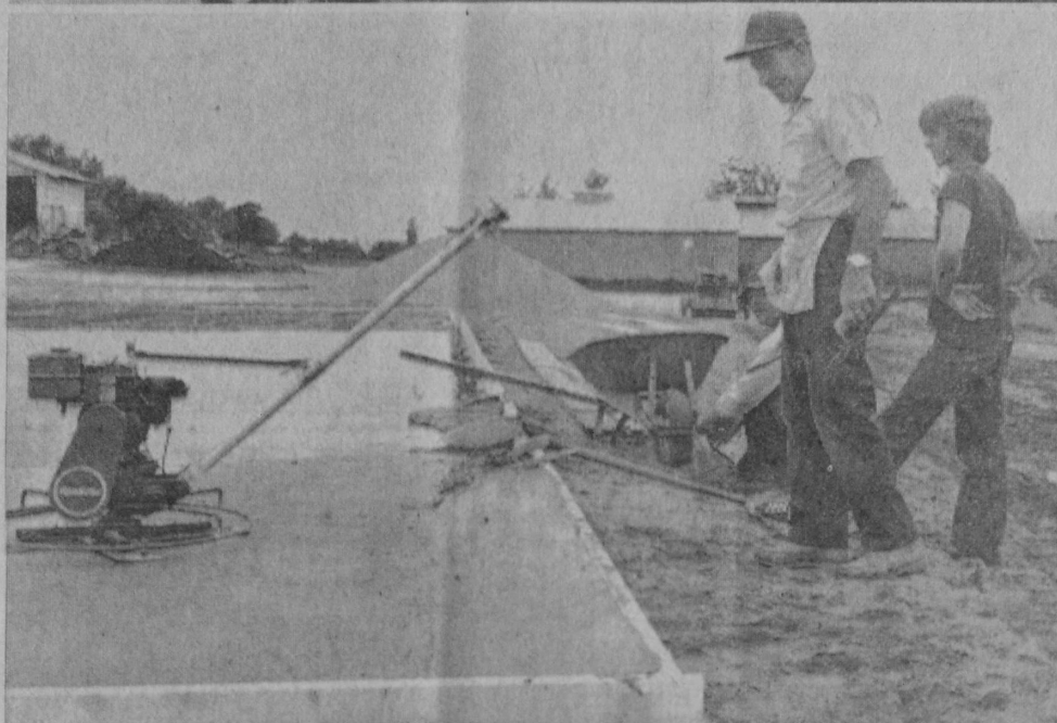
TAWAS RIVER mouth was much in the news during 1975, first when a sandbar completely blocked off the channel leading into Tawas Bay and later when dredging operations commenced, pictured at upper left. At lower left, volunteers constructed a new tennis court and ice skating rink at Hale through township funds
