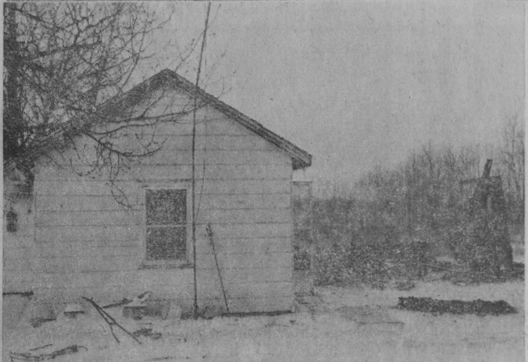
PLAINFIELD TOWNSHIP Fire Department answered two calls on Sunday, December 22. Fire gutted the frame home above owned by Mrs. Gerald Webb on Long Lake Road about 4:30 a. m. The home was not occupied at the time. The bottom picture shows all that remains of a snowmobile repair shop owned by Richard Eno on County Line Road south of Long Lake. A passing motorist turned in the alarm at 9:30 p. m. The building and contents were a complete loss.—Tawas Herald Photos.
