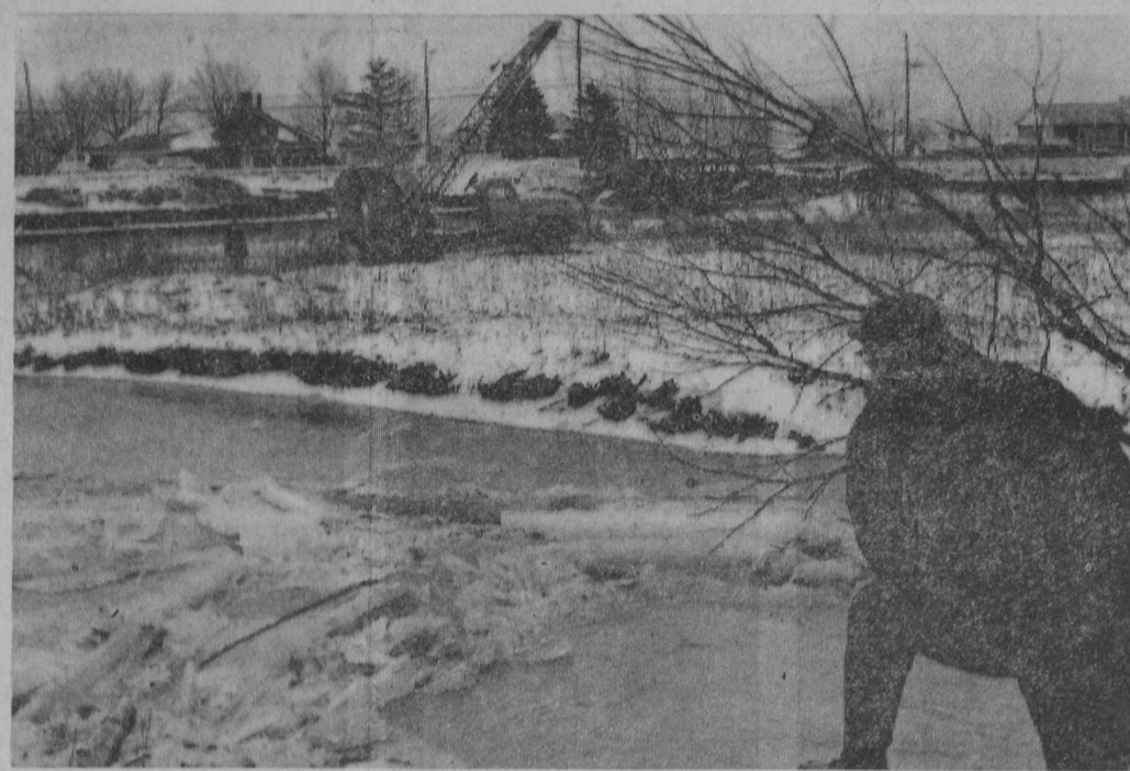
A SUDDEN THAW last January saw Dead Creek overflow its banks and caused a temporary flooding problem in Tawas City. The Tawas City Department of Public Works used its dragline to break up an ice jam. Flooding is again expected to be a problem in 1975.
