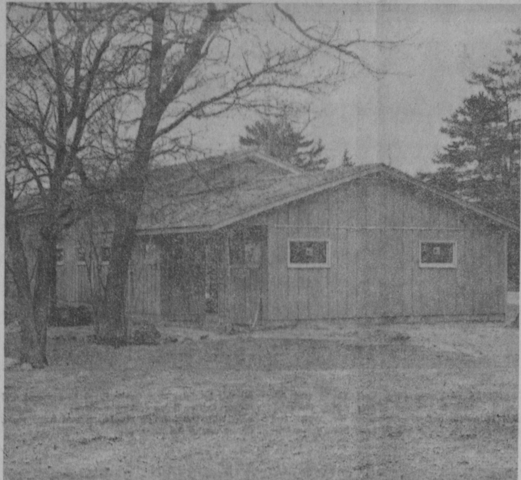
Work was started last year on a new headquarters for Tawas Point State Park.
