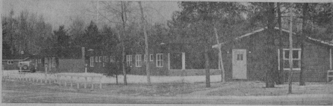
AMERICAN HOUSE-TAWAS AREA, a retirement village constructed in colonial rustic style at East Tawas, is nearing completion. One of the two-apartment carriage houses is at right and one of the four apartment wings in the lodge is shown in the center of the photo. —Tawas Herald Photo.
