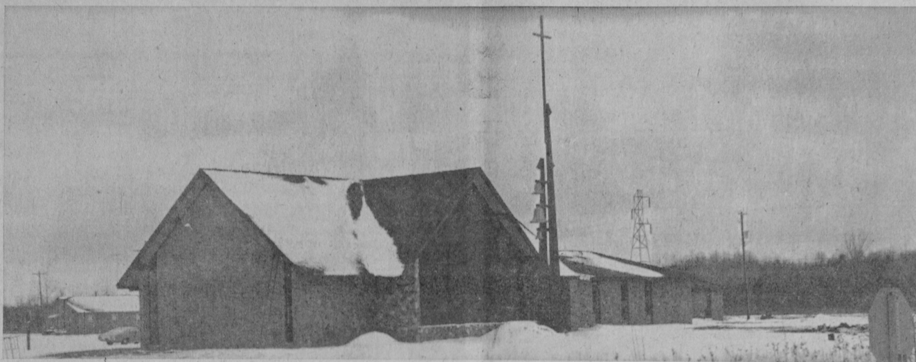
Looking at the new church from M-55
