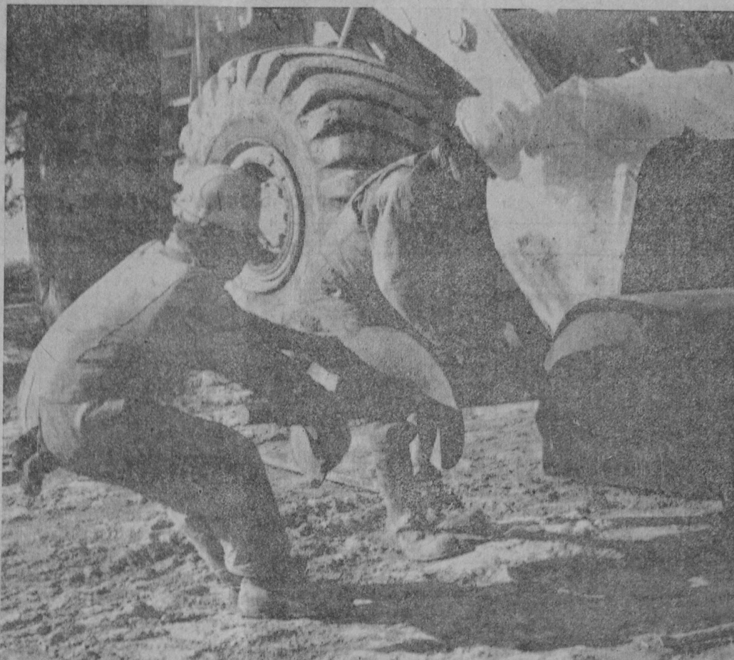
WORK WAS COMPLETED Thursday on boring under the Tawas River in sanitary sewer construction by T. A. Forsberg and Company. The main under the river is to connect with the lift station on First Avenue. This picture shows two workmen pulling the auger through a section of pipe.—Tawas Herald Photo.
