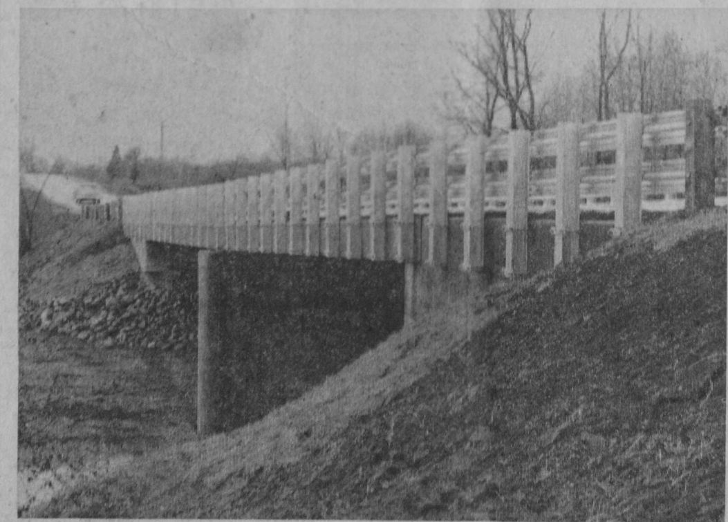
TRAFFIC on Whittemore Road between National City and Whittemore is now using this new $100,000 bridge which has been under construction since July. The bridge replaces an old iron truss structure which spanned the AuGres River for more than 40 years. During construction, traffic had been detoured to Turtle Road southwest of National City in order to meet M-65.—Tawas Herald Photo.
