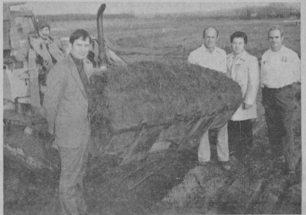
BREAKING GROUND for a new industrial building east of Whittemore took place Friday afternoon. Watching Hal Katterman operate the bulldozer are members of the Whittemore Industrial Development Corporation, from left: William McCluskey, treasurer; Paul Raynak, vice president; Henry Hicks, secretary, and Albert (Bud) Wrathell, president.—Tawas Herald Photo.
