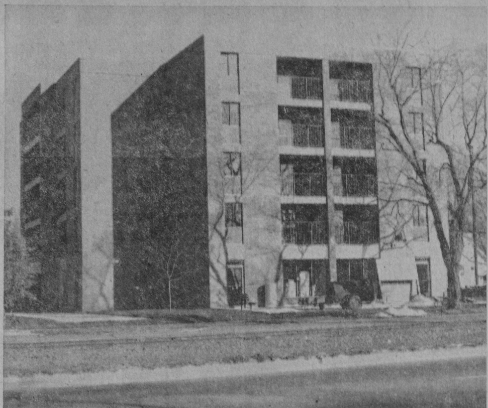
THE BEAUTIFUL new high rise apartment building on Bay Street at East Tawas is nearing completion. No announcement
