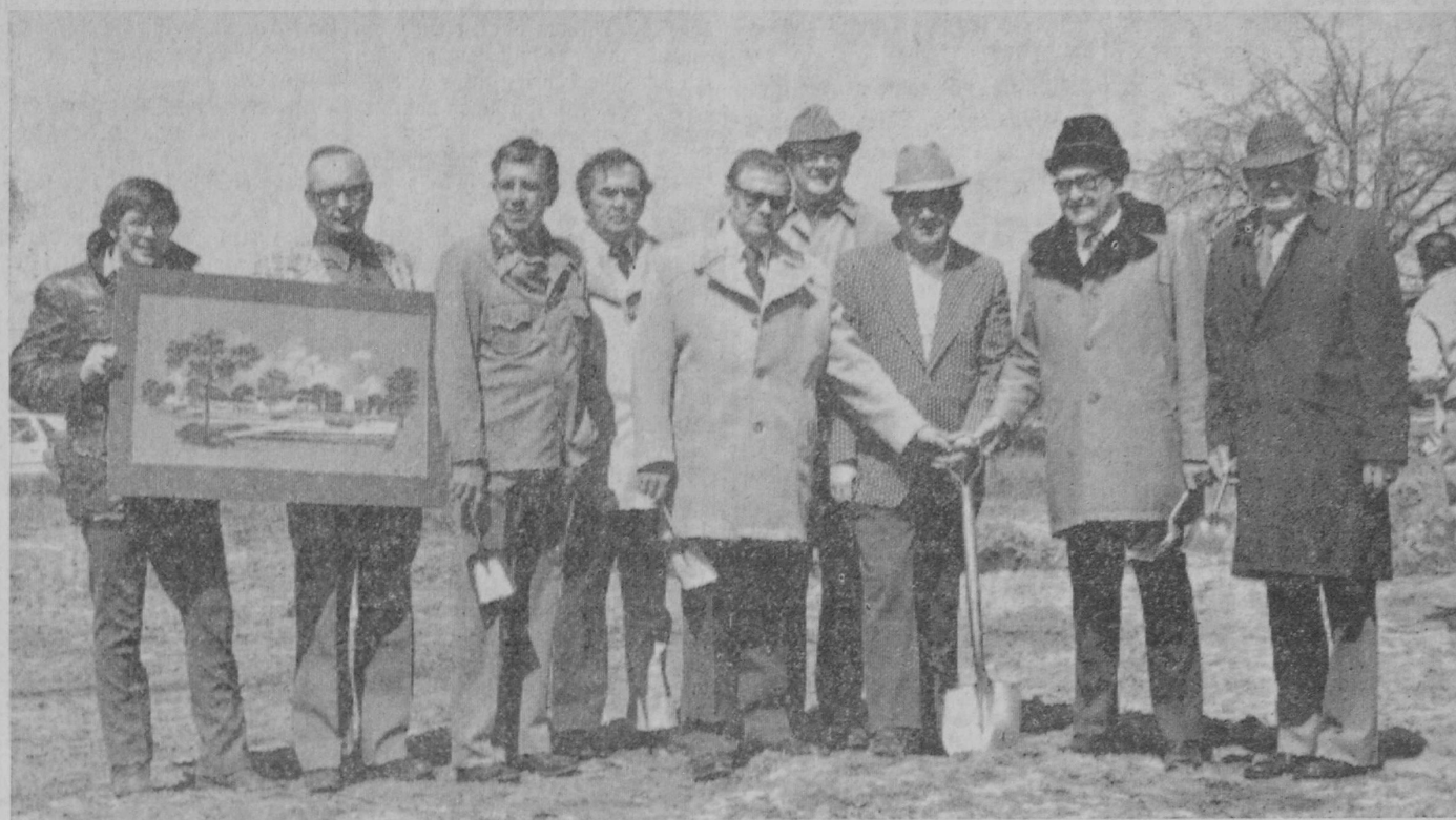
PARTICIPANTS in Thursday's ground breaking ceremony for the new Iosco County Road Commission garage on M-55 are pictured above. From left are James Delahanty, county road commission engineer-manager; Douglas Basel, architect, Scott Engineering Company; William Wereley, county commissioner; Donald Griffin, county commissioner; Robert Foster, chairman of the county board of commissioners; Joseph Fox, county commissioner; Merton Killely, chairman of the county road commission; Henry M. Conley, county road commissioner; Arthur Aulerich, county road commissioner.—Tawas Herald Photo.
