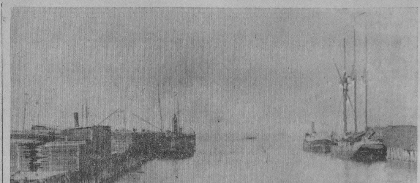
THE MOUTH of the AuSable River is pictured here in the early 1890s at about the end of the major lumbering industry, which peaked in 1891. Manufactured lumber is piled on docks awaiting
