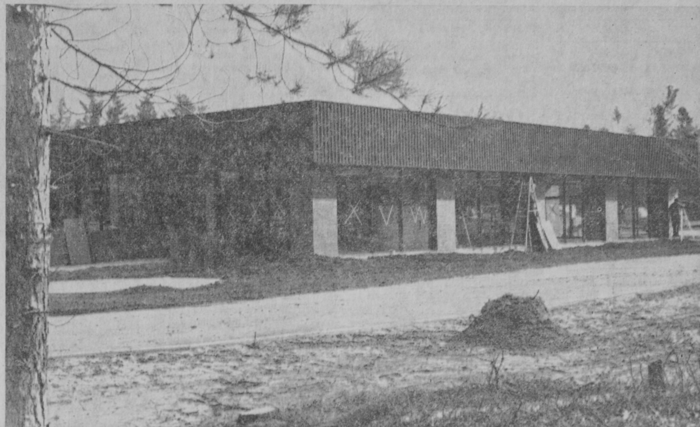
NEW SHOWROOM of McIntosh-McKay Chevrolet-Cadillac was being readied Monday morning for the grand opening to be held Friday, Saturday and Sunday. The 26,000-square foot building has been under construction since last August.—Tawas Herald Photo.
