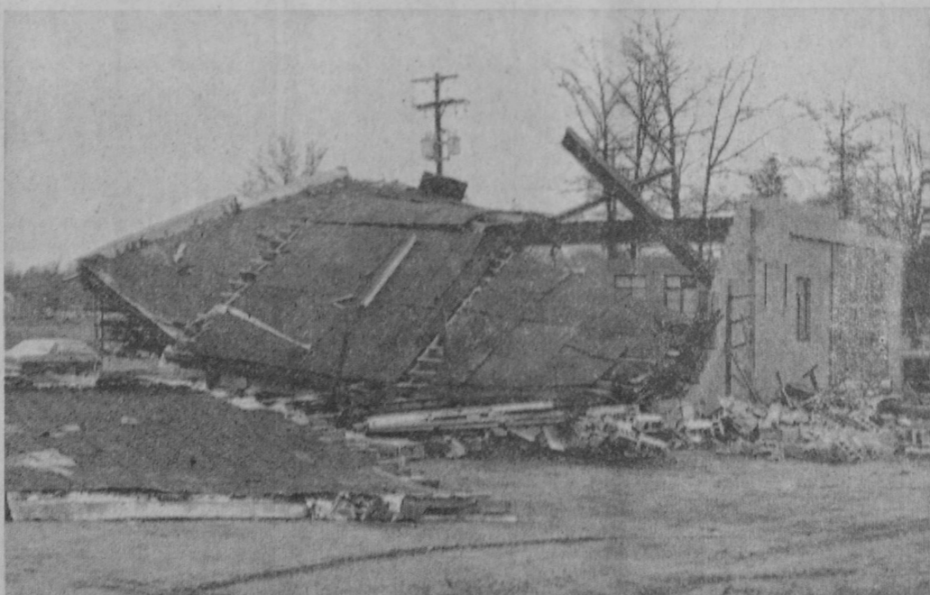
THIS COMMERCIAL BUILDING owned by James Quigley, located on the Ogemaw County side of South Branch, was demolished when the twister touched down March 30. One mobile
