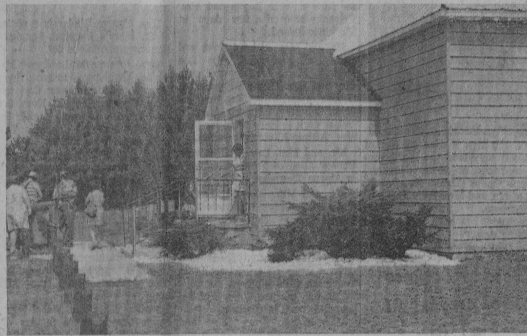
RECENTLY REMODELED Burleigh Township Hall is pictured above. The old building on Putnam Road was renovated as a centennial project during the nation's bicentennial year using manpower provided by CETA. The township was organized in May 1876.—Tawas Herald Photo.
