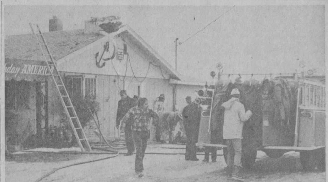
TAWAS CITY FIREMEN battled a blaze Saturday noon in frigid weather at Coyle's Restaurant. The fire was confined to the kitchen area and the roof. Flames damaged an exhaust system in the kitchen which vented out of the roof of the building.—Tawas Herald Photo.
