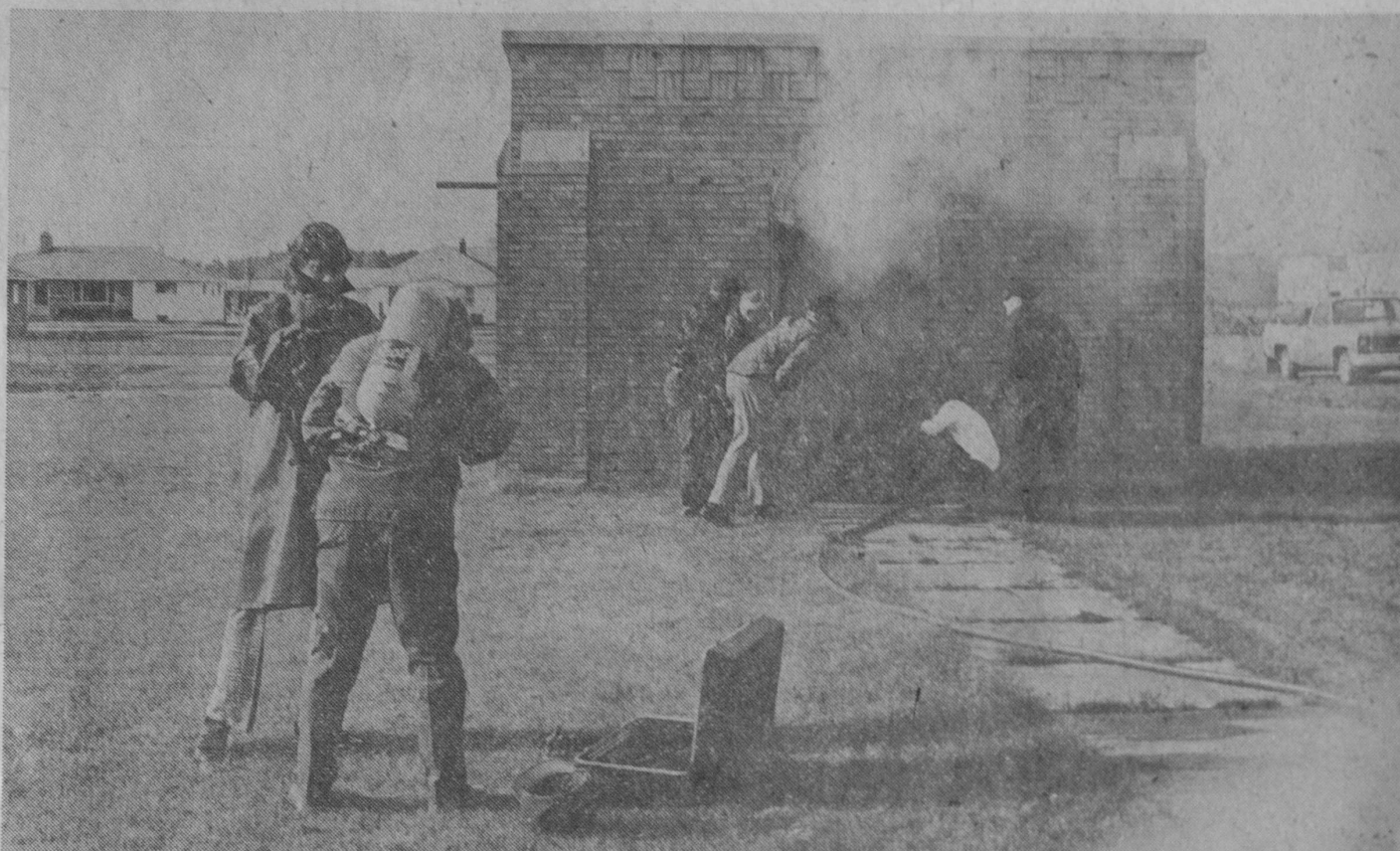
TAWAS CITY'S deep well pumping station on First Avenue was knocked out of commission for a little more than an hour Wednesday noon when a fire damaged the installation's electrical power service. Although firemen were not positive as to the exact cause of the blaze, it was believed that a heating unit in the building was responsible. "We were fortunate that pumping equipment and the electric motor were not damaged and the station was out of service for only a short time," said City Mgr. Reginald Bublitz. Be-
