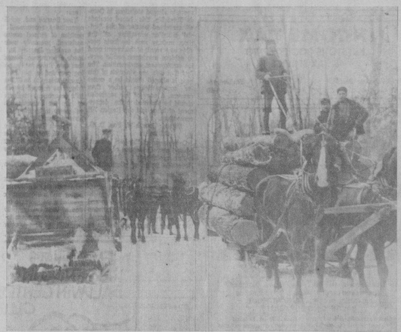
EIGHTY YEARS AGO in Plainfield Township, road construction took place during winter months! The roads were different than today's network of asphalt paving—then, they had a surface of ice for a specialized purpose. Heavy loads of saw logs could not be moved by brute strength alone and all the skills of an experienced teamster were required. After carefully packing snow on a road with a roller, a special tanker sleigh was used to sprinkle water on the surface of the road. The work was usually done at night when the water would freeze almost instantaneously when it hit the surface. The result was a smooth, slick road of solid ice, upon which sleighs piled high with logs could be easily pulled by a team of horses, especially shod to travel on the slick surface. When the road began to wear out, a new application of water renewed the surface.
