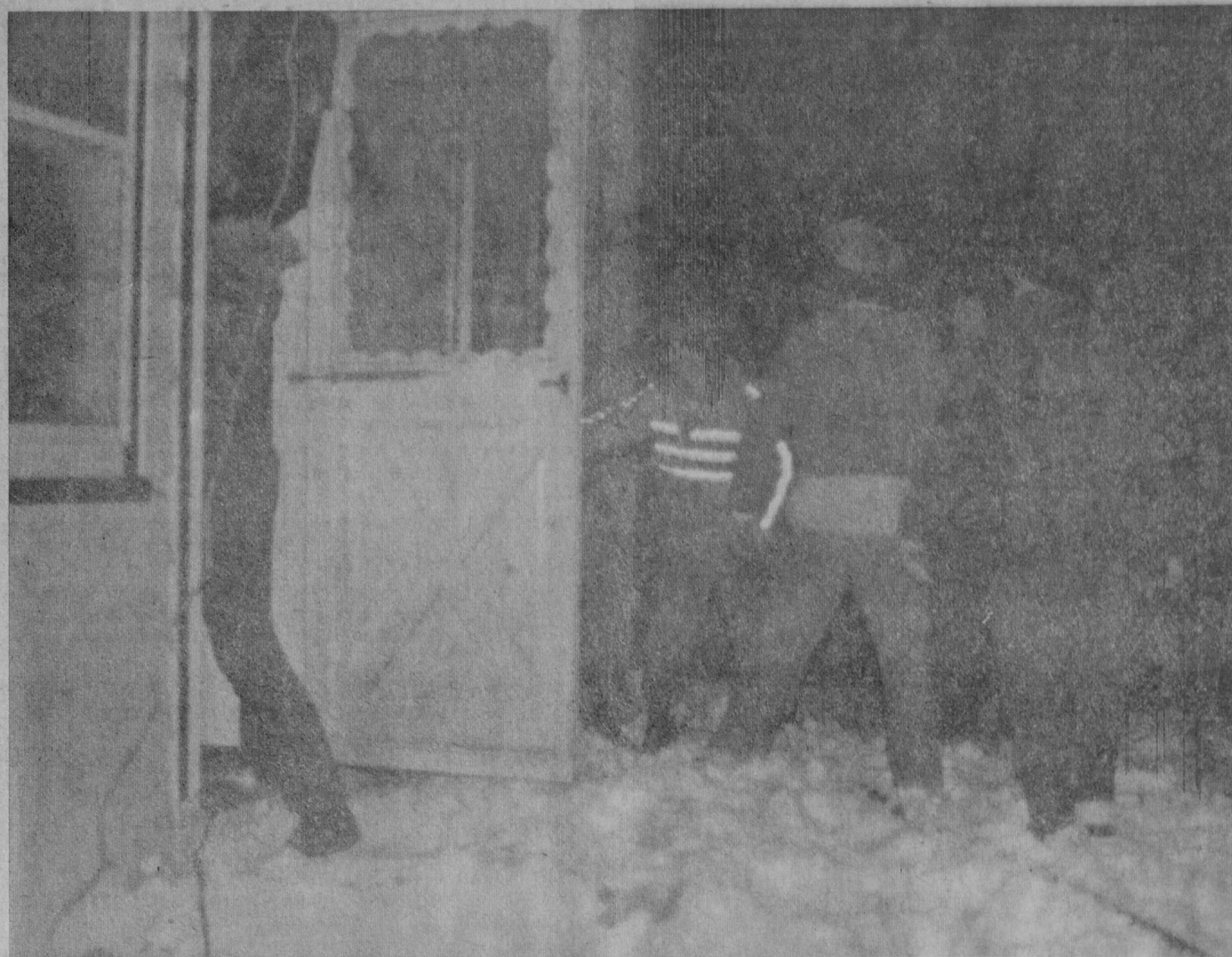
TAWAS CITY FIREMEN were called on two blazes over the weekend. The first fire was reported Saturday night at the residence of Mr. and Mrs. David Fisher on Meadow Road. A fire, believed to have started in a bedroom closet, caused extensive damage to the
