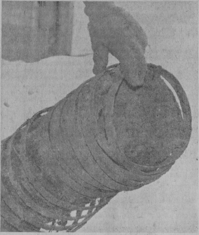
A SECTION of the iron banded wooden pipe which once conveyed salt brine from East Tawas to AuSable-Oscoda is pictured here. —Tawas Herald Photo.
