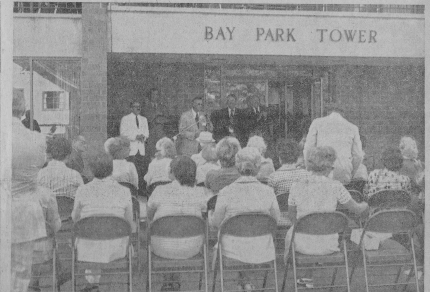
FORMAL DEDICATION and open house at Bay Park Tower, a high rise housing unit for the elderly at East Tawas, was held Saturday afternoon. Toastmaster for the outdoor ceremony was John C. Elliott, president of the East Tawas Housing Commission, shown at the microphone. Other speakers included Cong.
